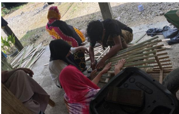
Figure 14. Trash bin construction together with residents
